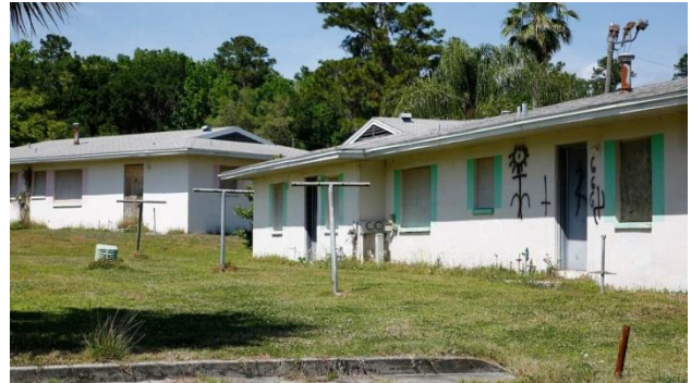
Housing units that once housed low-income families in Brooksville at Hillside Estates have been abandoned for years. At the urging of the U.S. Department of Housing and Urban Development, the Brooksville Housing Authority recently accepted a bid for purchasing the development.
