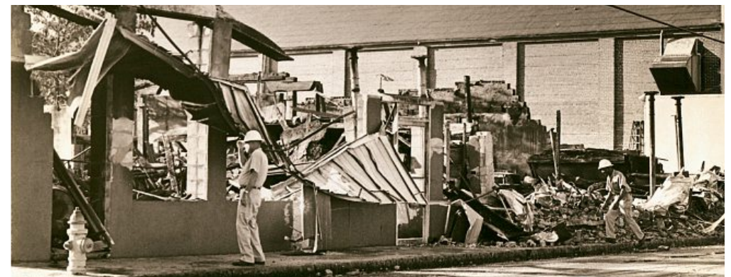
Work got underway to clean up the debris left behind by days of looting and rioting near Central Avenue after the shooting of Martin Chambers in 1967. Times (1967)
