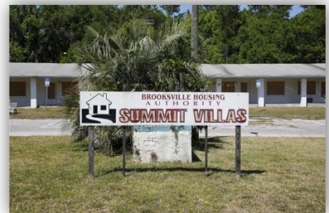
LUIS SANTANA | Times --Brooksville Housing Authority's Summit Villas is boarded up and abandoned.
