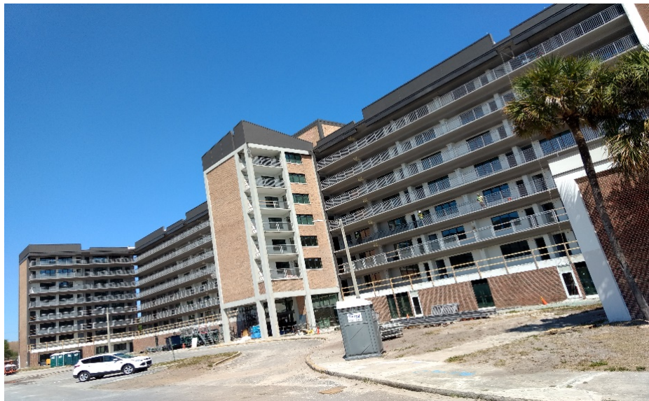
ABOVE: T2A MARY BETHUNE IN PROGRESS
