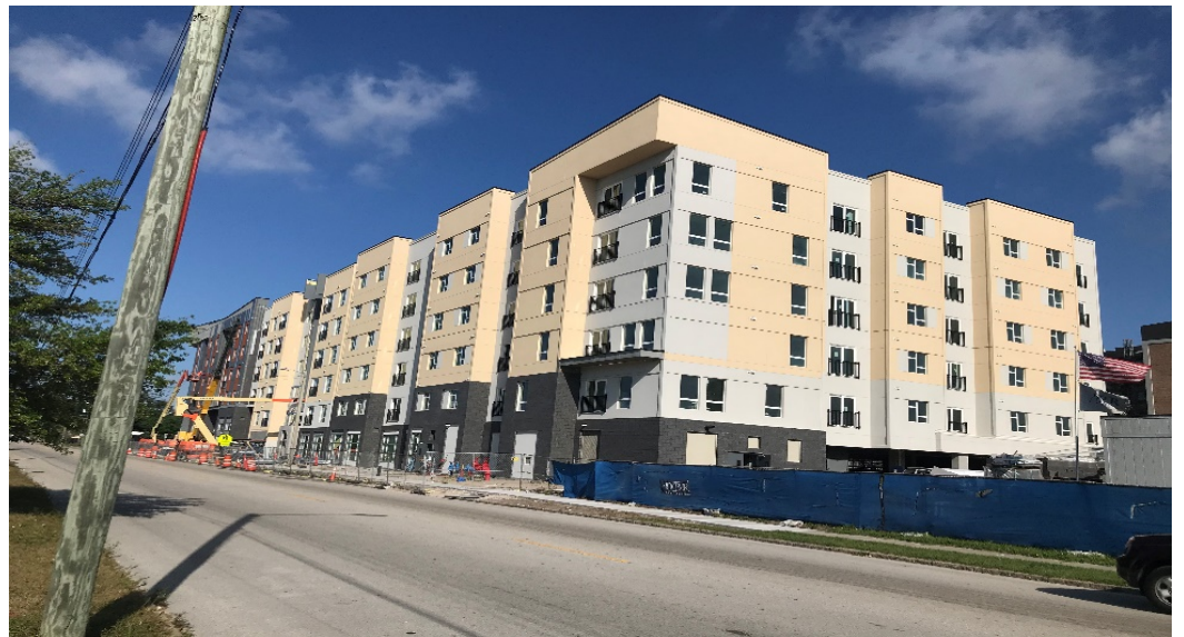
ABOVE: T-1 RENAISSANCE AT WEST RIVER IN PROGRESS
