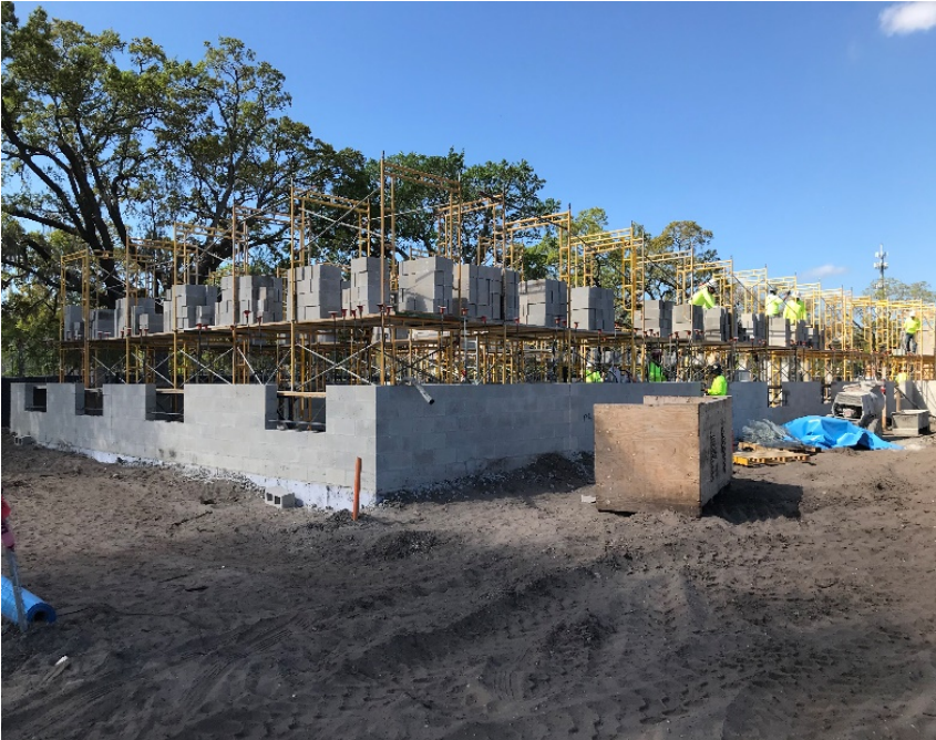
ABOVE: T3A IN PROGRESS
