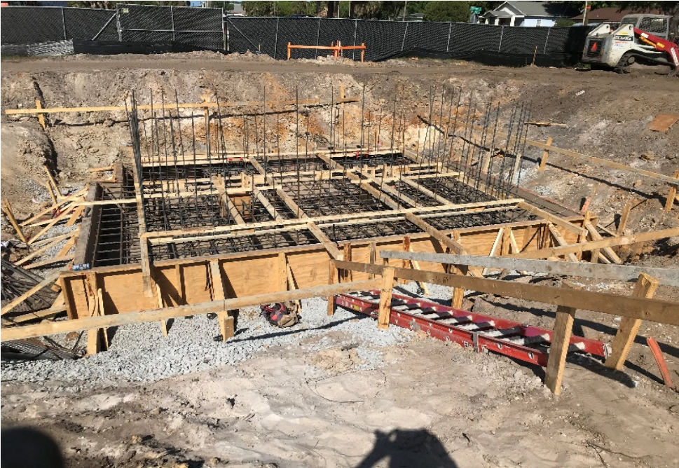
ABOVE: T3C- IN PROGRESS
