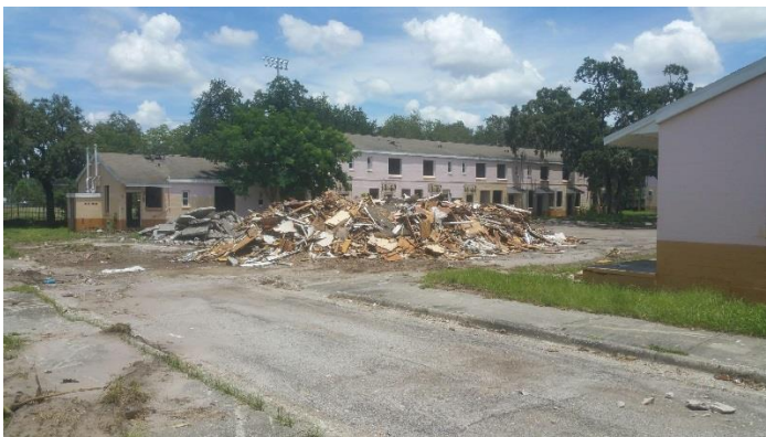
NBH Demo Phase 2 underway.
