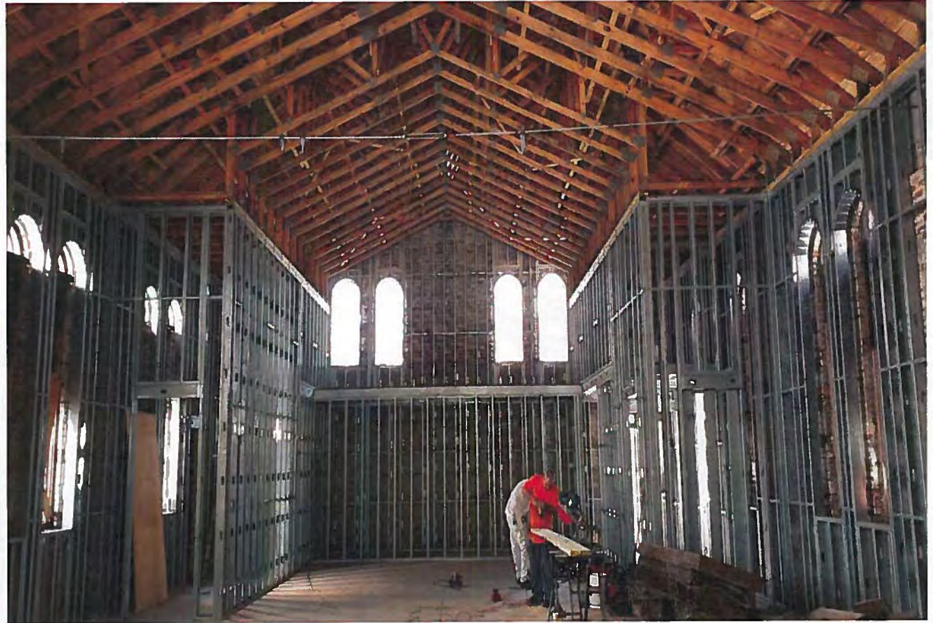
Church Interior Framing
