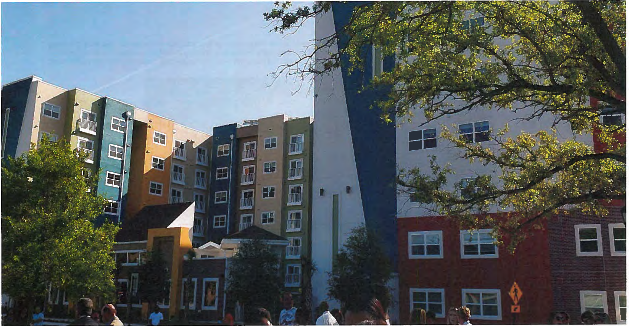
Tempo – Construction is complete. In Close-out Phase. 203 Units -199 Occupied.
