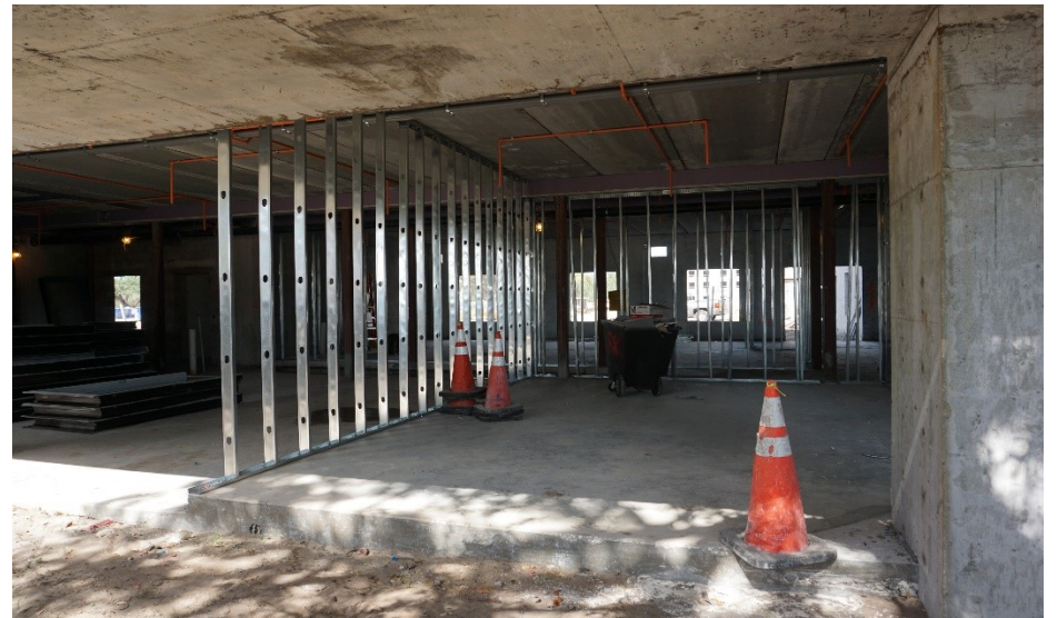
Interior Unit Framing in Progress (A Different View)
