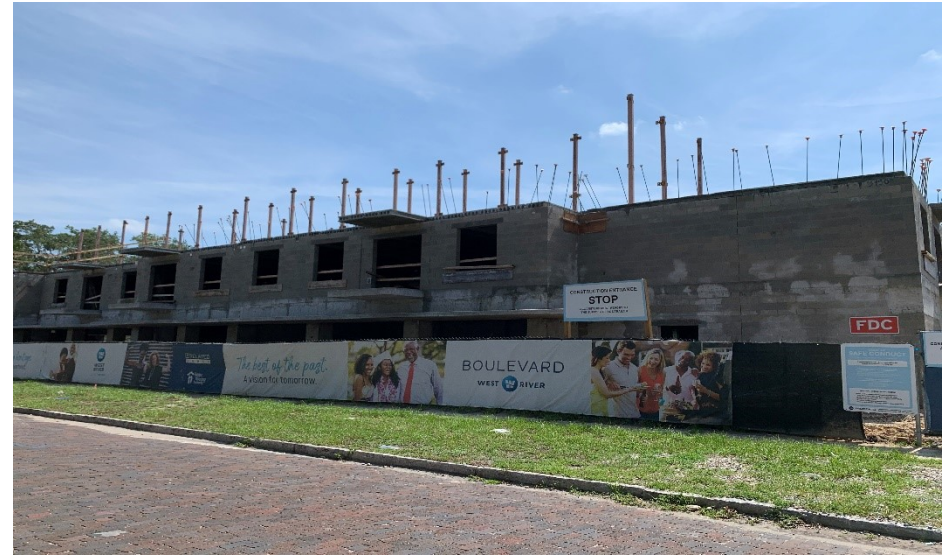
Tower 2 Exterior Walls Front View in Progress
