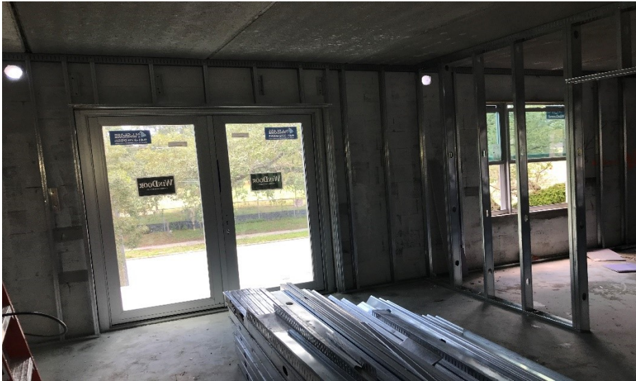
Interior Framing in Progress
