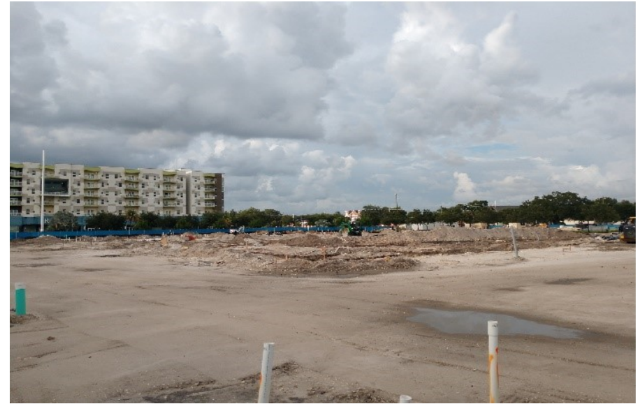
Legacy - Site Grading In Progress
