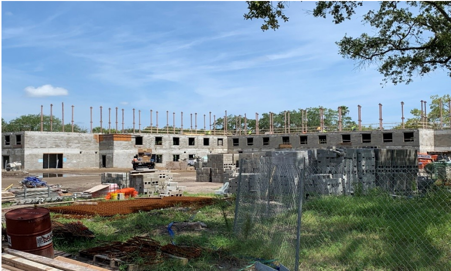
Tower 2 Exterior Walls in Progress
