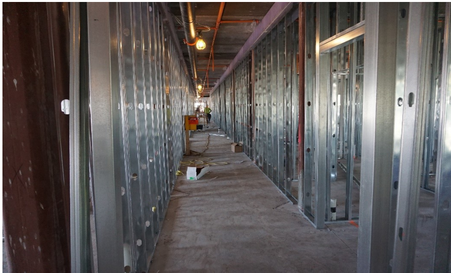
Typical Hallway Framing in Progress
