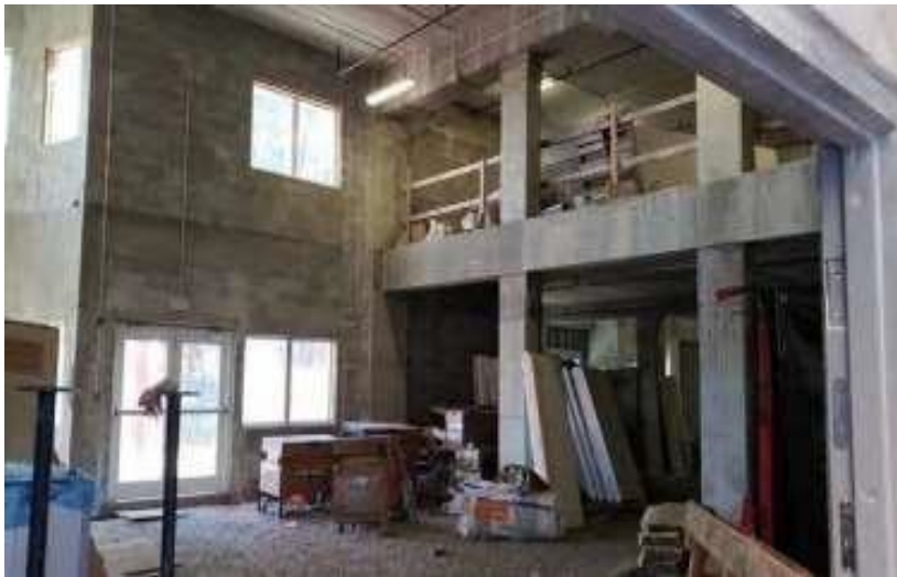
Theatre Interior Pending
