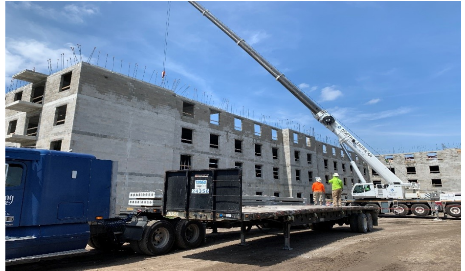
Hollow Core Plank Installation in Progress
