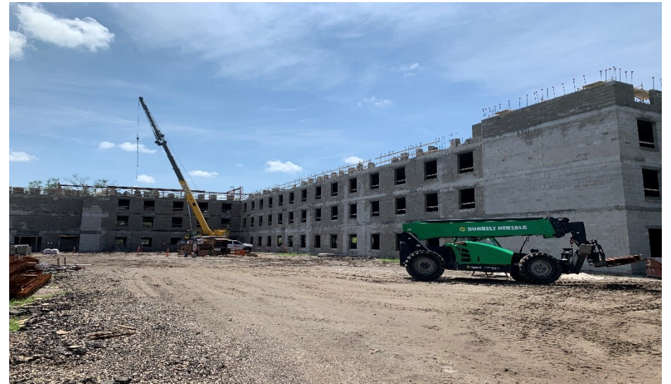
Tower 3 Hollow Core Plank Installation in Progress
