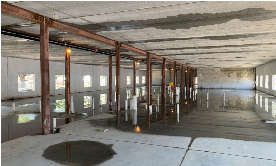
Tower 2 View of Interior Space and Hallway in Progress
