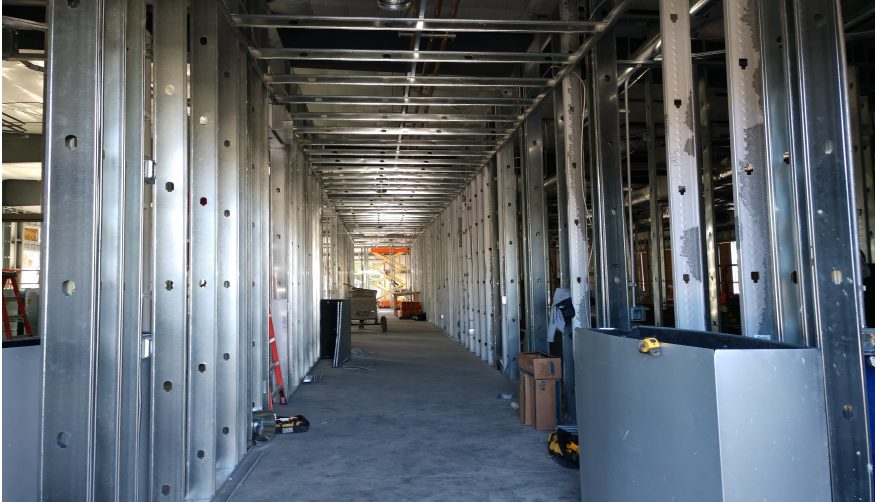
Project currently under construction, utilities added to building slab, and foundation complete. Building is topped out. Roof complete. Interior metal framing has begun and MEP ( Mechanical Electrical Plumbing). Rough-end has started. Completion scheduled January 24th, 2020.
