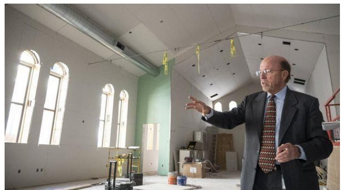
David Hollis with the Tampa Housing Authority tours renovation work under way at the St. James Episcopal Church. Built in 1921, St. James was once a hub for the community known as The Scrub. [JAMES BORCHUCK | Times]
