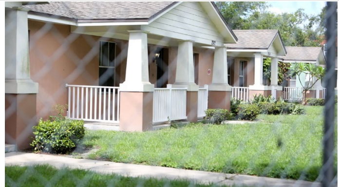
The bungalows at Jordan Park in St. Petersburg sit empty behind a gate put up to enclose the properties. Federal money to rehabilitate the public housing project is in jeopardy. [MARTHA ASENCIO RHINE | Tampa Bay Times]
