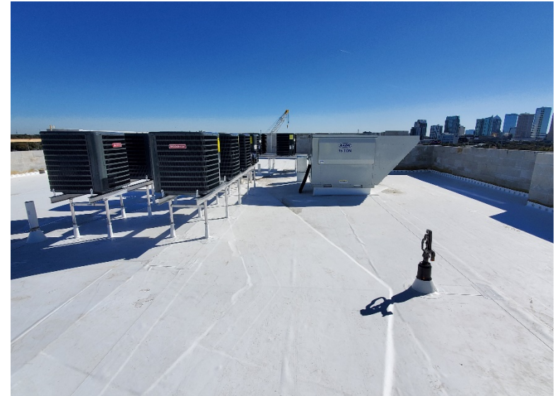
Tower 1 – Roof A/C Compressor Install in Progress
