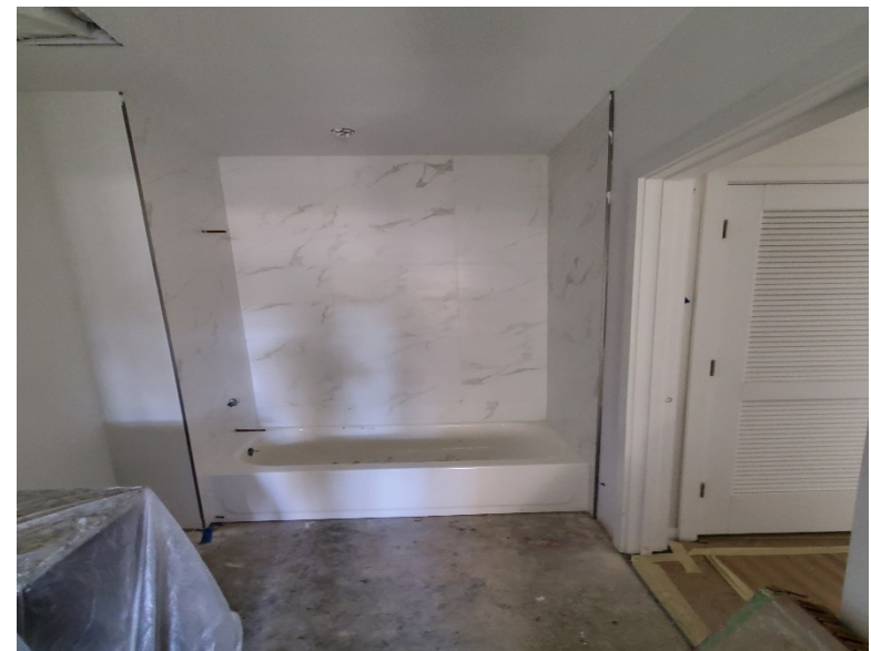
Tower 1 – 7 th Floor Bathtub Install in Progress
