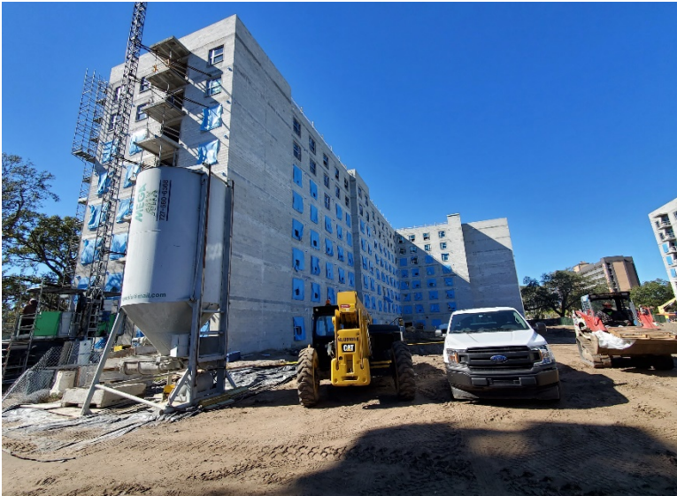
Tower 1 – Exterior Elevation in Progress
