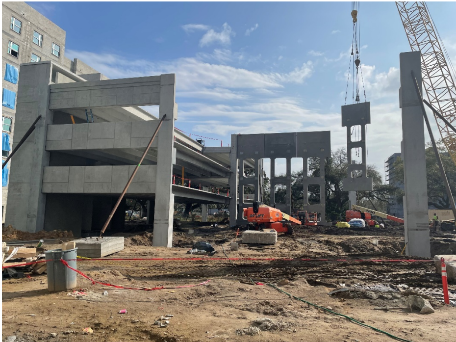
Garage 1 – Vertical and horizontal pre-manufactured conc panels install in Progress
