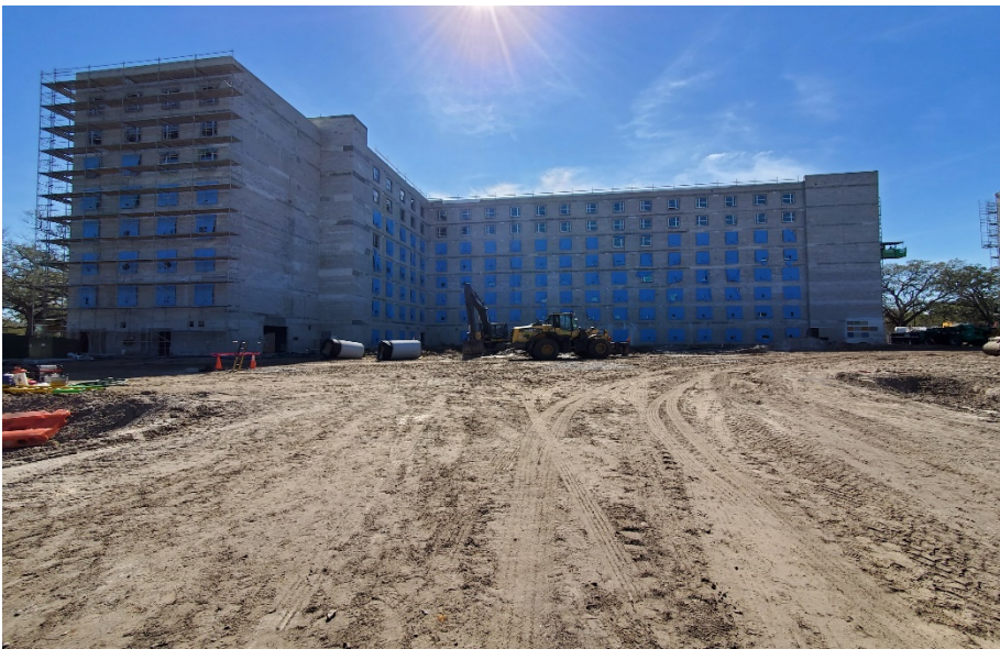
Tower 3 – Exterior Elevation in Progress
