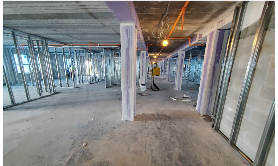
Tower 2 – 6 th Floor Wall/Ceiling Framing Install in Progress
