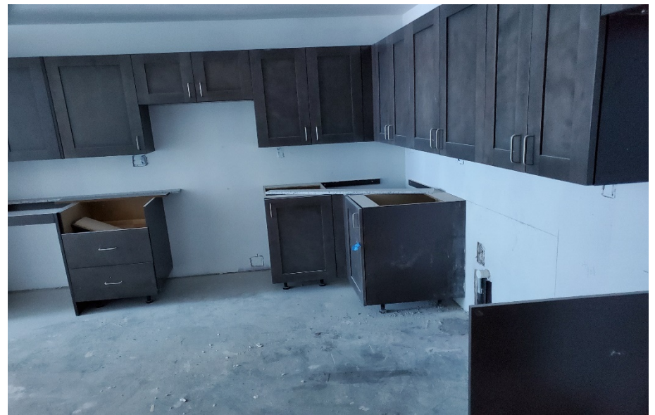
Tower 3 – 3 rd Floor Kitchen Cabinets Install in Progress
