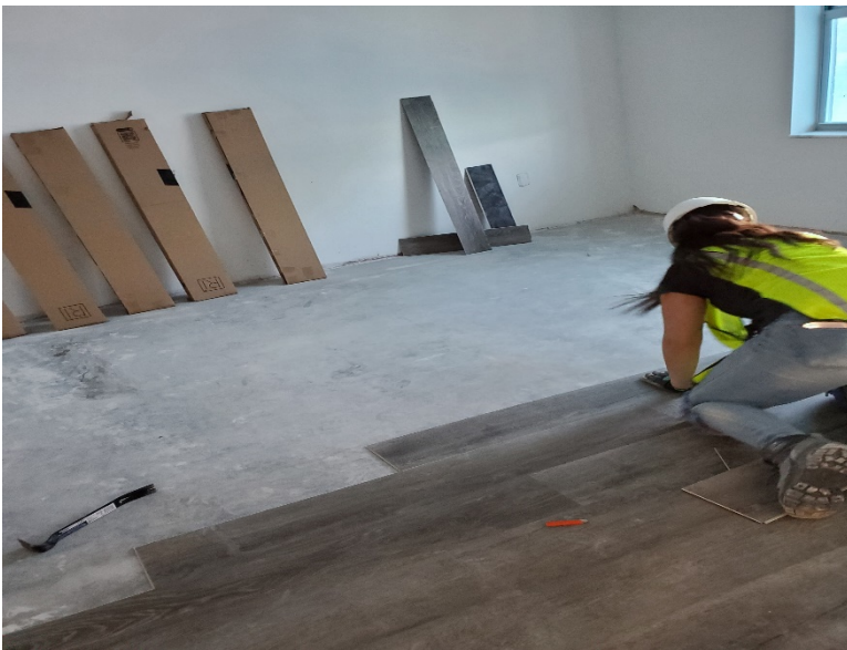
Tower 1 – 2 nd Floor Flooring Install in Progress
