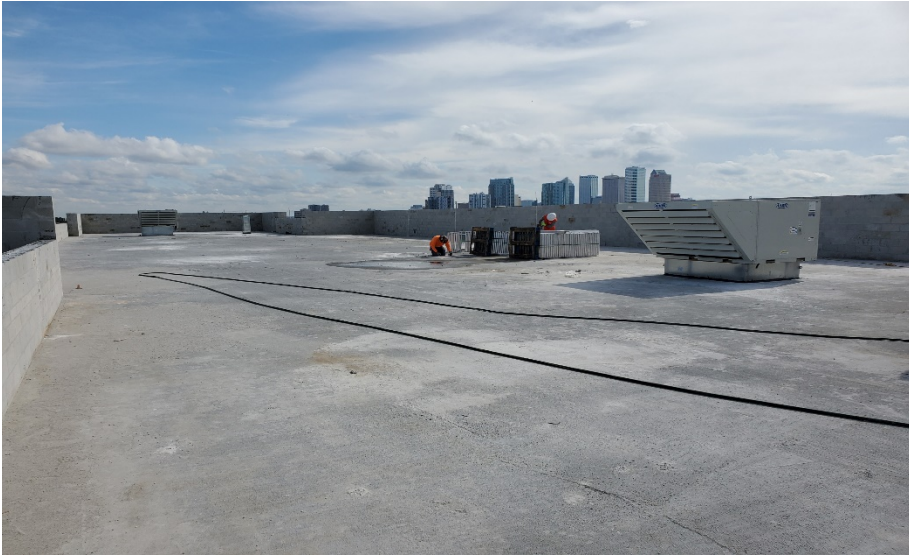
Tower 2 – Roof Install and MEP Rough-in in Progress
