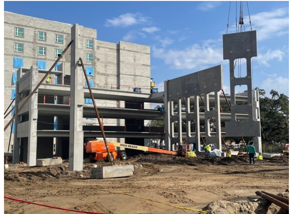
Garage 1 – Vertical and horizontal pre-manufactured conc panels install in Progress
