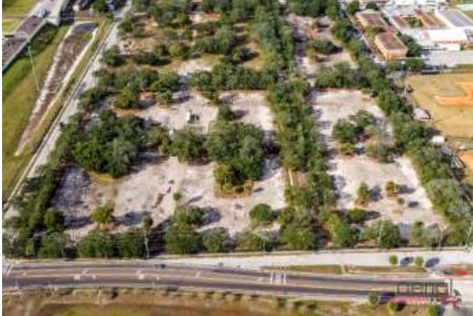
NBH Demo Phase 2 underway.
