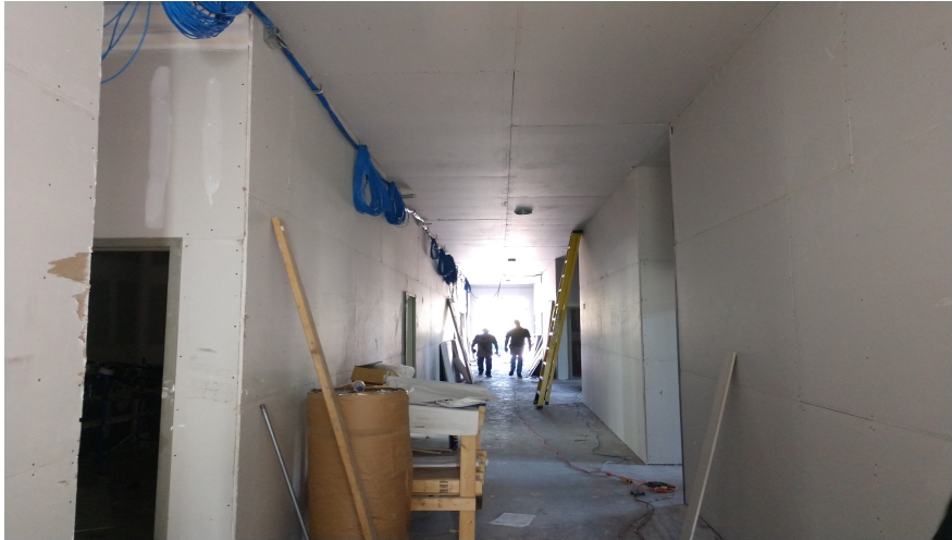
Project currently under construction, utilities added to building slab, and foundation complete. Building is topped out. Roof complete. Interior metal framing is complete and MEP ( Mechanical Electrical Plumbing) final is being installed. Interior Drywall 75% complete Completion scheduled February 2020.
