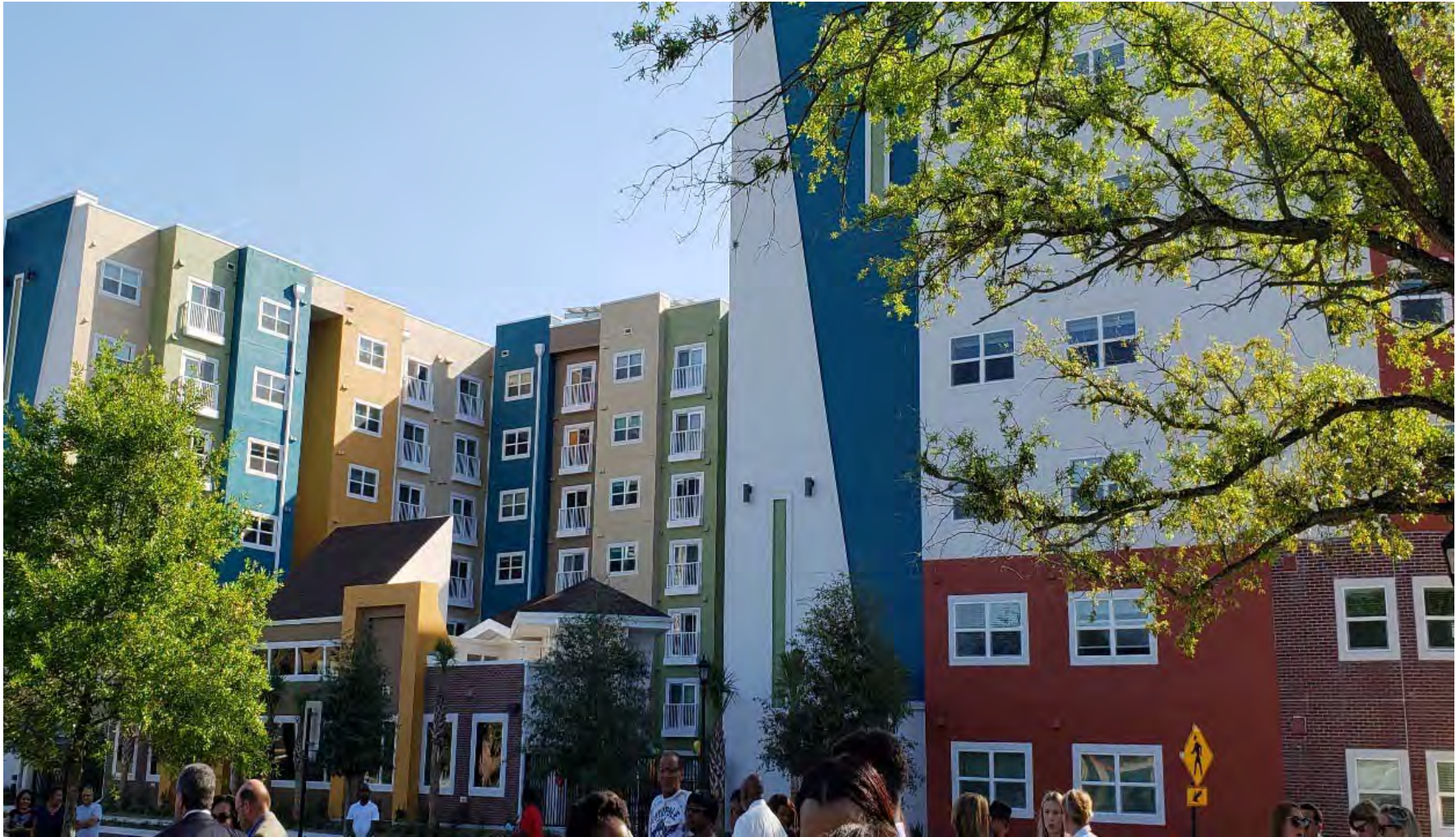
Tempo – Construction is complete. In Close-out Phase. 203 Units -199 Occupied.
