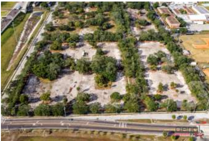
NBH Demo Phase 2 underway.
