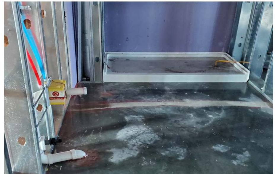
Tower 3 – 4th Floor Shower Pans Install in Progress
