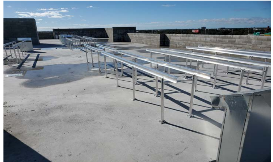
Tower 1 – Roof Install in Progress
