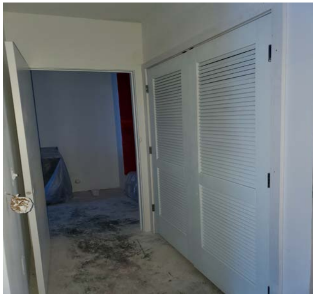
Tower 1 – 1st Floor Apartment Doors Install in Progress
