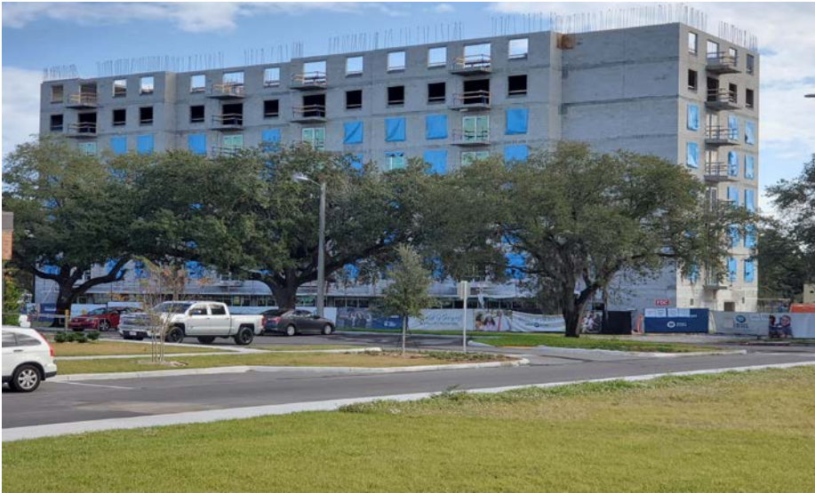
Tower 2 – Exterior Elevation in Progress
