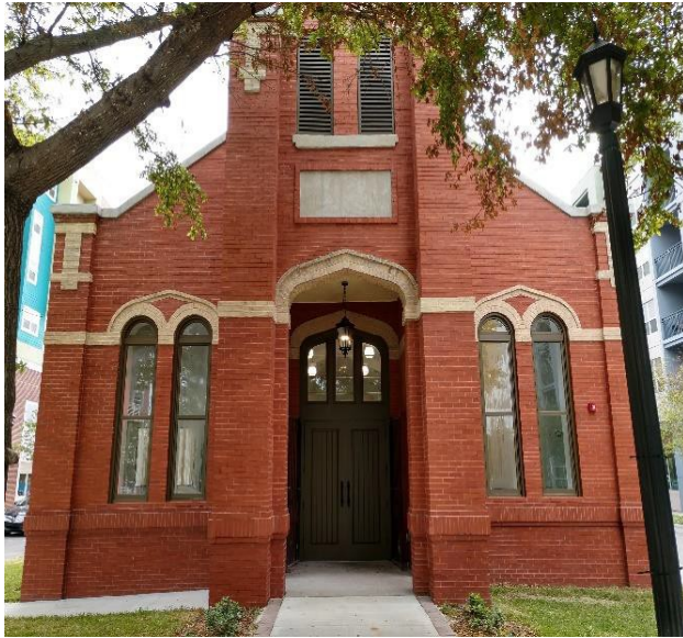
Front doors and glass transom now fully restored, per City of Tampa Historic Preservation ARC requirements.
