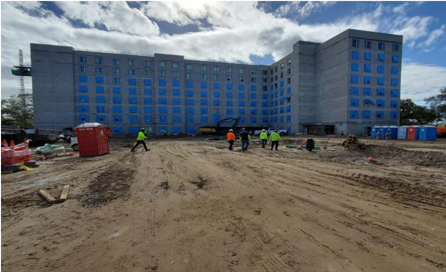
Tower 1 – Exterior Elevation in Progress
