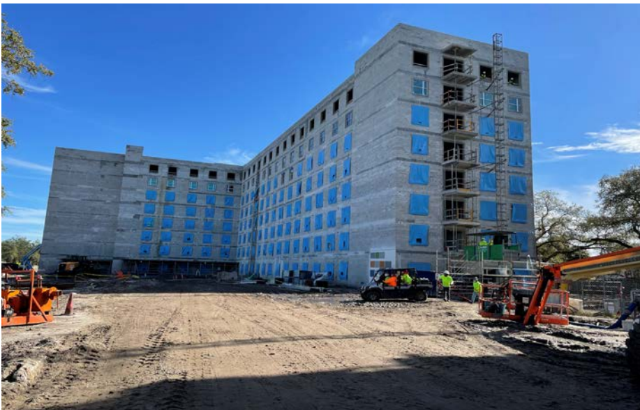
Tower 3 – 8 th Floor Windows Install in Progress
