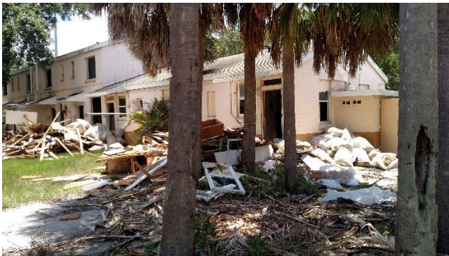
NBH Demo Phase 2 underway.
