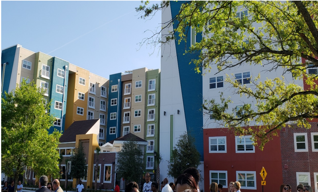
Tempo – Construction is complete. In Close-out Phase. 203 Units -196 Occupied.
