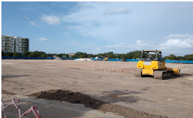
Lot 11 – Site grading in progress
