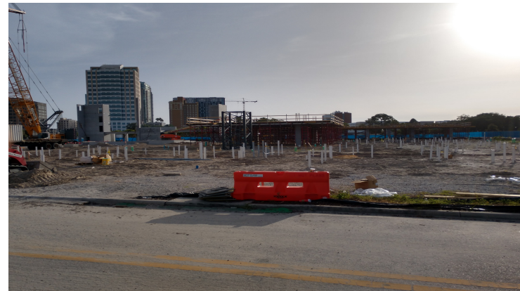
Lot 9 underground utilities and support columns
