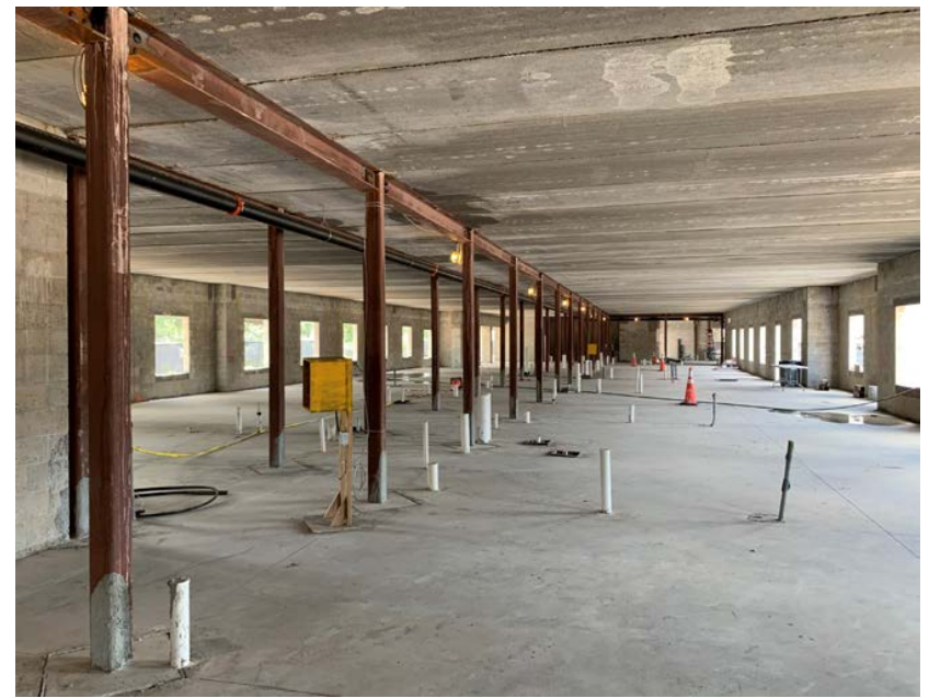
T3A 1 st CEILING AND FRAMING
