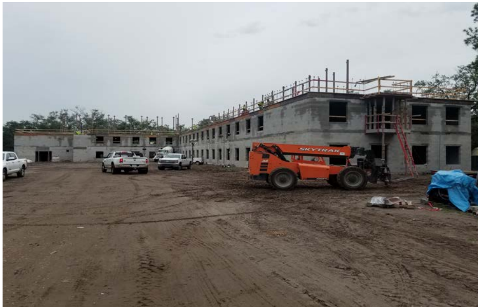
T3B 2 ND FLOOR PERIMETER WALLS INSTALLED
