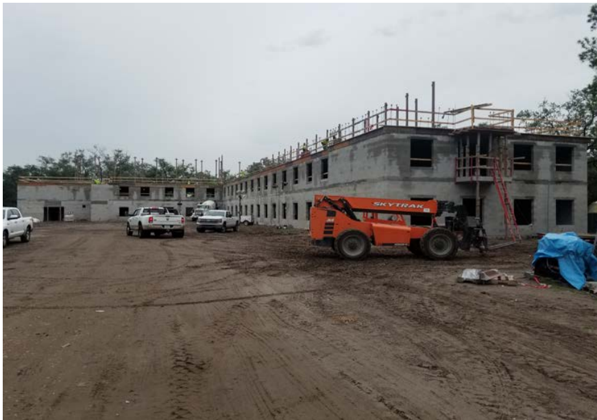
T3B 2 ND FLOOR PERIMETER WALLS INSTALLED
