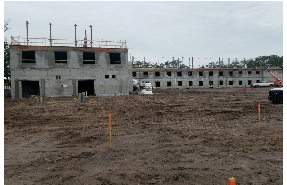
T3C EXTERIOR CONCRETE BLOCK WALLS, 2 ND FLOOR
