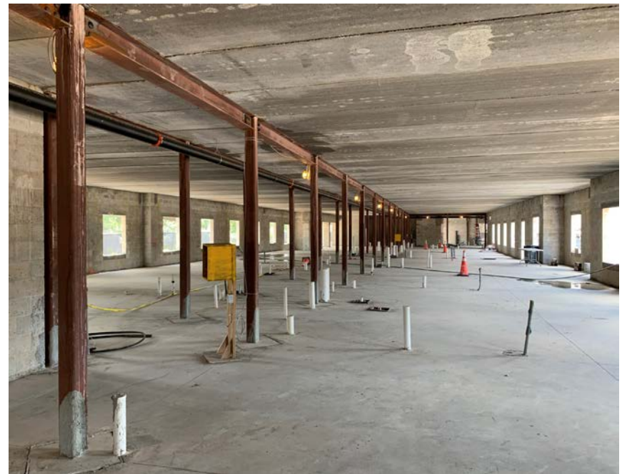
T3A 1 st CEILING AND FRAMING
