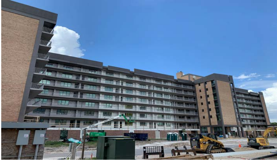
Below: Mary Bethune Hi Rise Building
