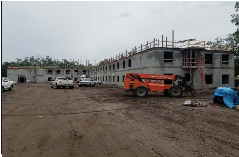
T3B 2 ND FLOOR PERIMETER WALLS INSTALLED
