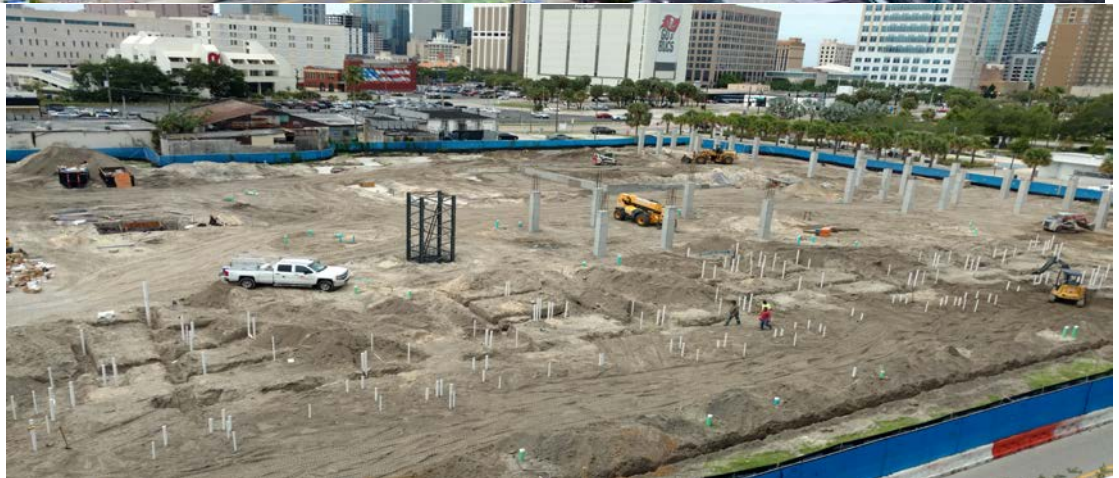
Lot 9 underground utilities and support columns
