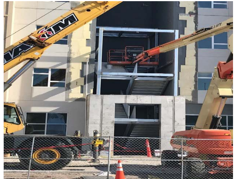
Above: Renaissance in construction phase
