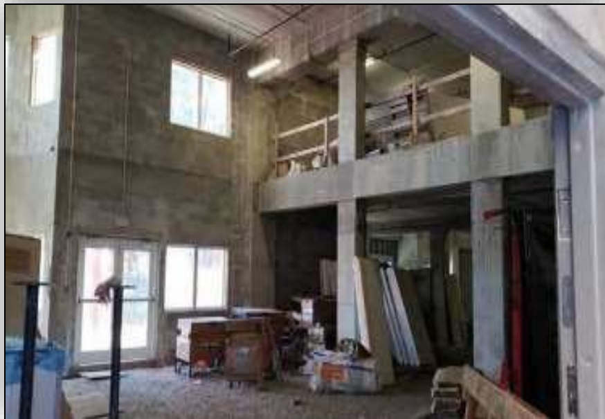
ABOVE: THEATRE INTERIOR
