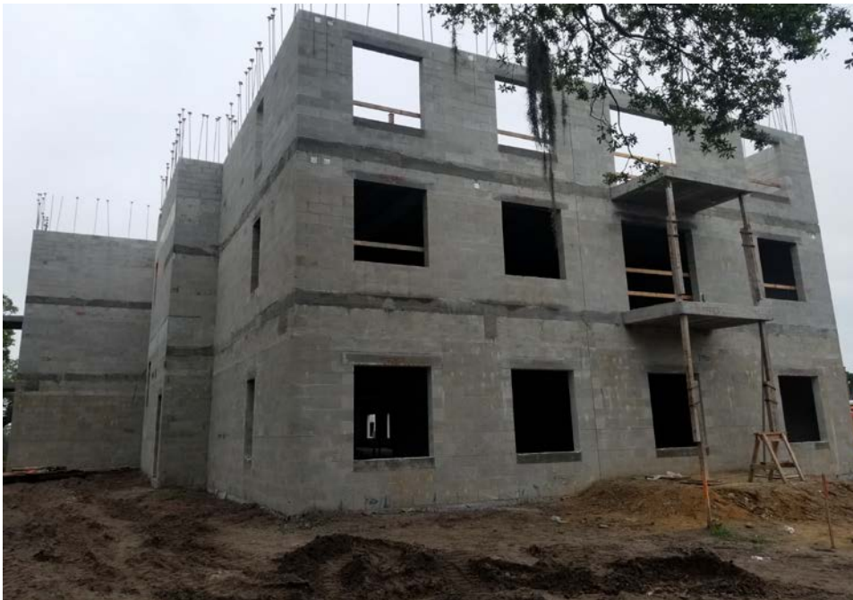
T3A- PERIMETER WALLS BEING INSTALLED
