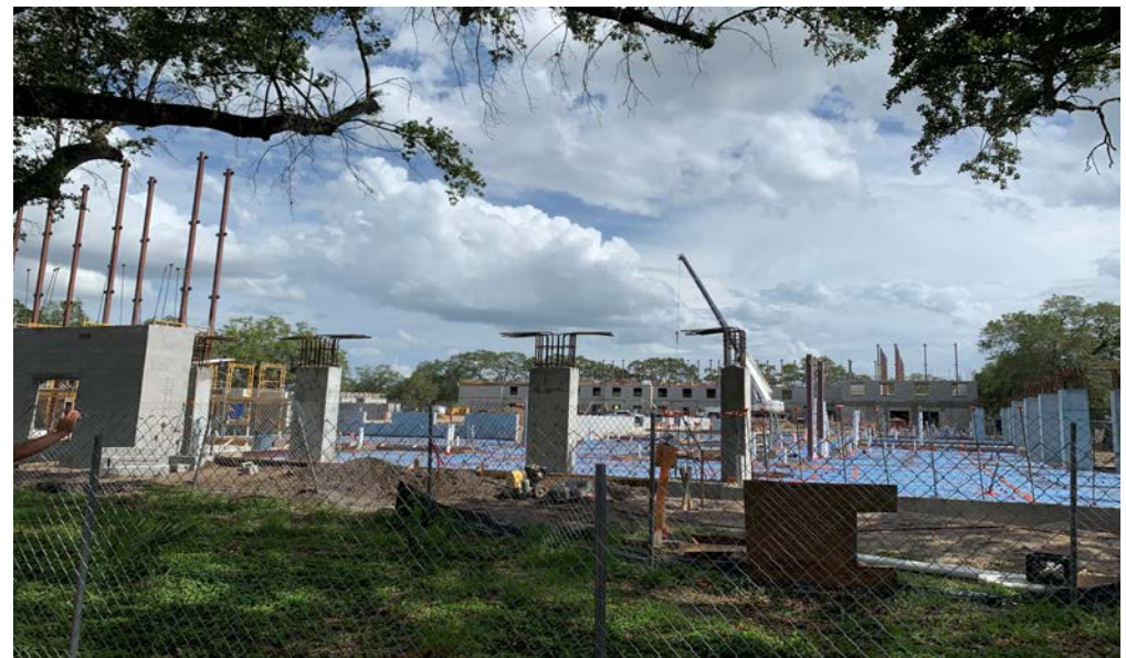
T3C PAD, FOOTER AND 1 ST FLOOR WALLS
