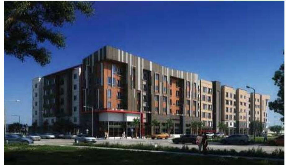
T1- The Renaissance at West River- 160 Senior Housing units
