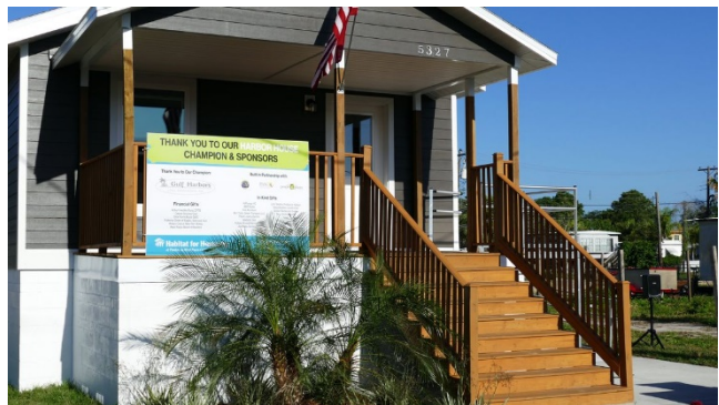
1MICHELE MILLER | Times In 2019, Habitat for Humanity of Pinellas and West Pasco counties celebrated the completion of the 'Harbor House' in Town and Country Villas in New Port Richey. The neighborhood is part of Habitat's West Pasco revitalization initiative to bring affordable housing to the New Port Richey area. Last week, Pasco commissioners said they will waive transportation fees for new single-family and multifamily affordable housing projects. [CT BOWEN | Tampa Bay Times]
