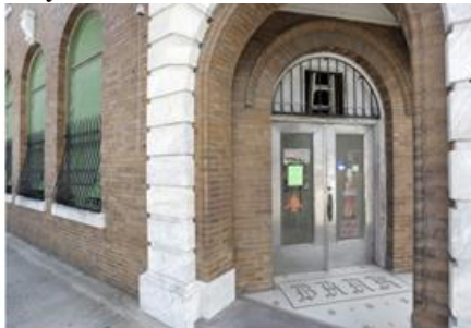
Figure 5 --The Fourth of July Cafe closed in June. Once a staple of Main Street, it operated out of the old Bank of West Tampa building on the corner of north Howard Avenue. West Main Street in west Tampa was once a thriving economic boom for African-Americans and Cuban-American businesses. [OCTAVIO JONES | Times]
