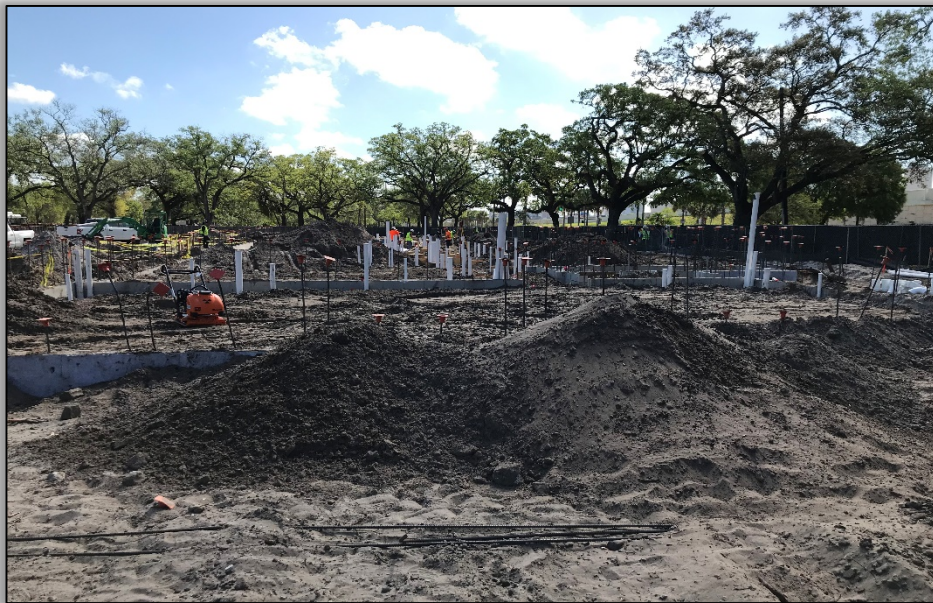
T3B FOUNDATION WALLS INSTALLED
