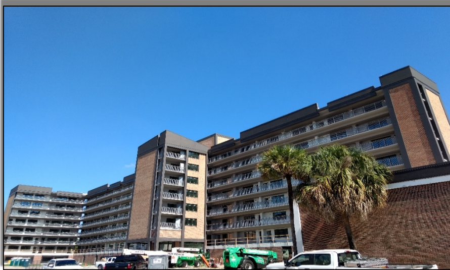
Below: Mary Bethune Hi Rise Building
