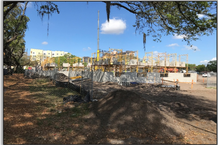
T3A- PERIMETER WALLS BEING INSTALLED
