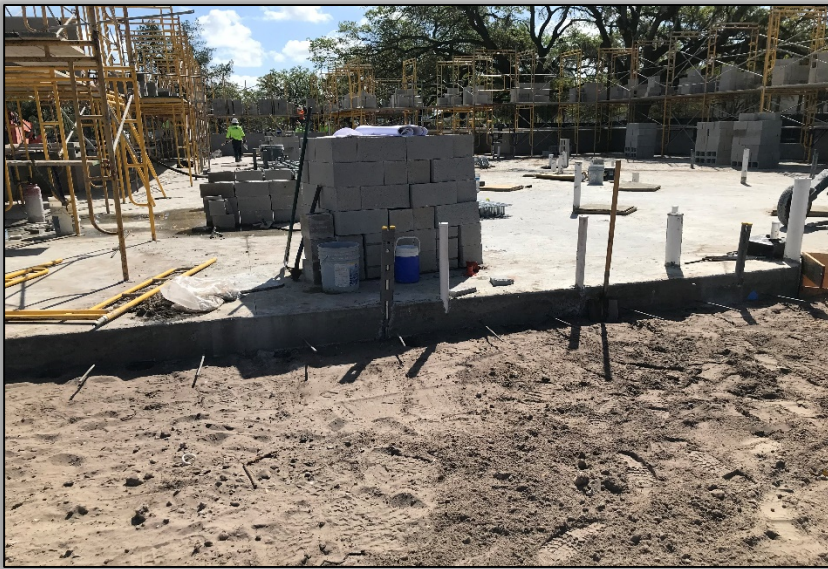
T3A-CONCRETE PADS INSTALLED
