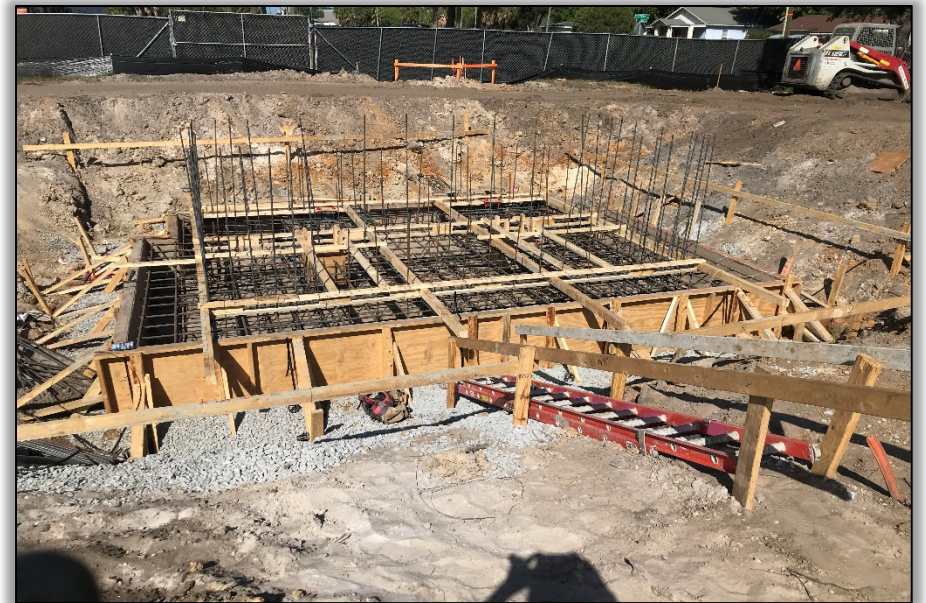
T3C PAD & FOOTER FORMED INSTALLED
