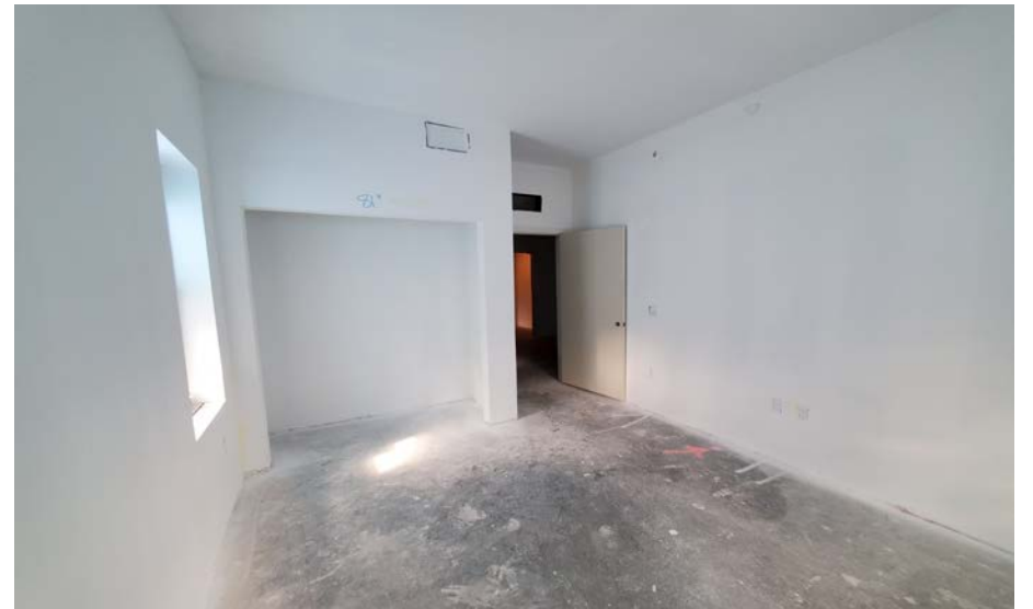
Tower 1 – 1 st Floor Interior Wall Paint Priming in Progress
