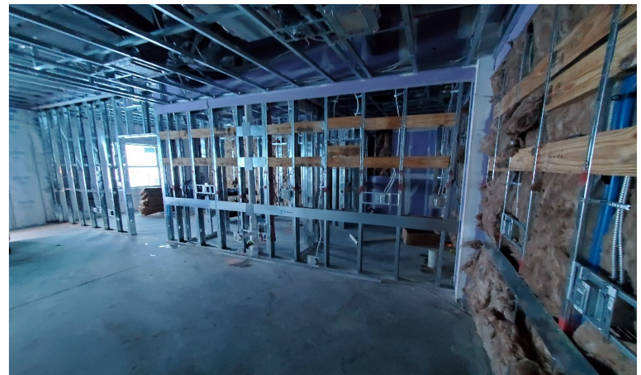
Tower 3 – 4 th & 5 th Floor Interior Wall Framing in Progress
