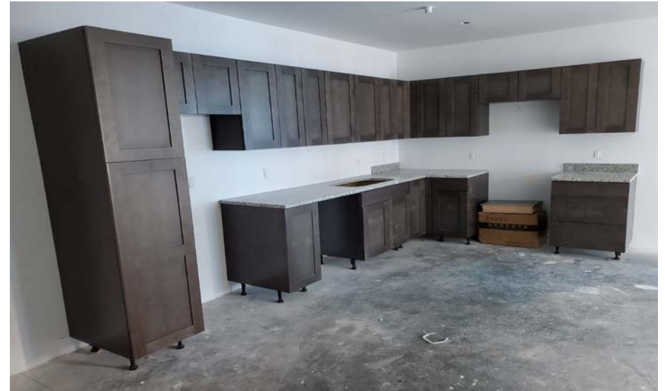
Tower 1 – 1 st Floor Interior Unit Kitchen in Progress
