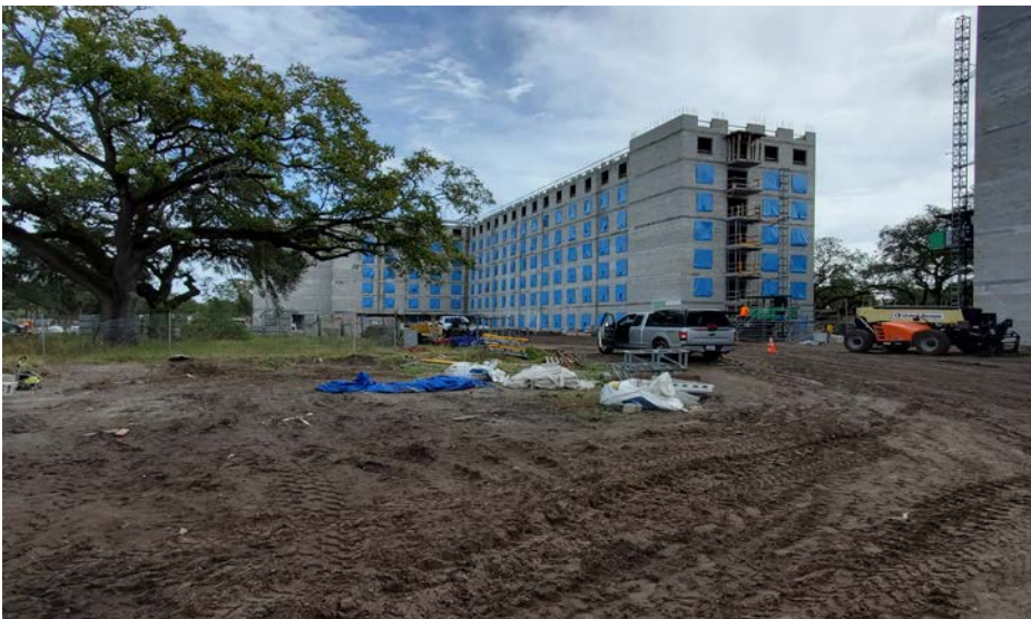
Tower 3 – 8 th Floor Hollow Core Plank Install in Progress
