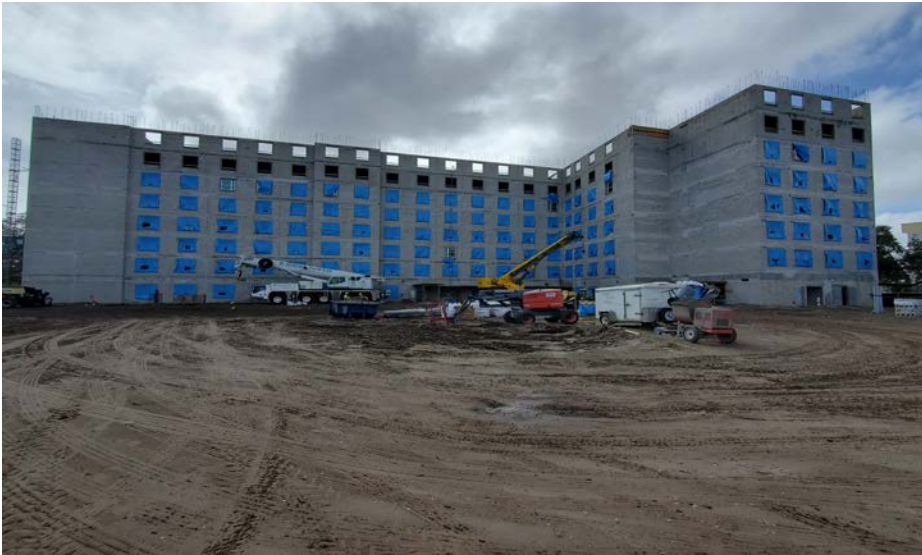
Tower 1 – 8 th Floor CMU Walls install in Progress
