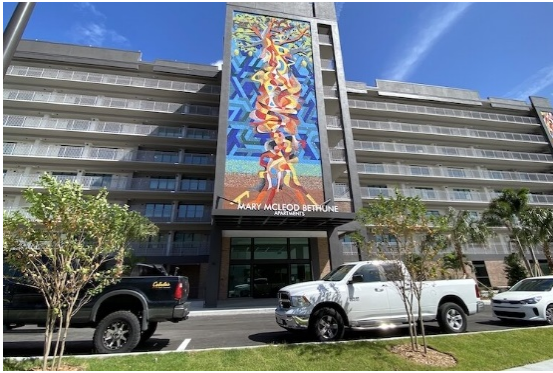
Courtesy of Tampa Housing Authority Hennessey Construction renovated the Mary McLeod Bethune building, with Place Architects as designers.
