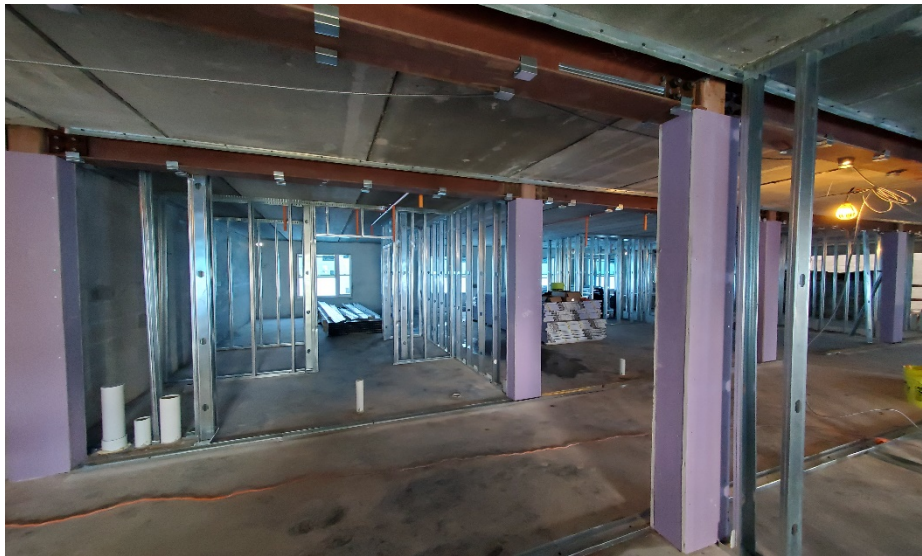
Tower 1 – 5 th Floor Interior Wall Framing in Progress
