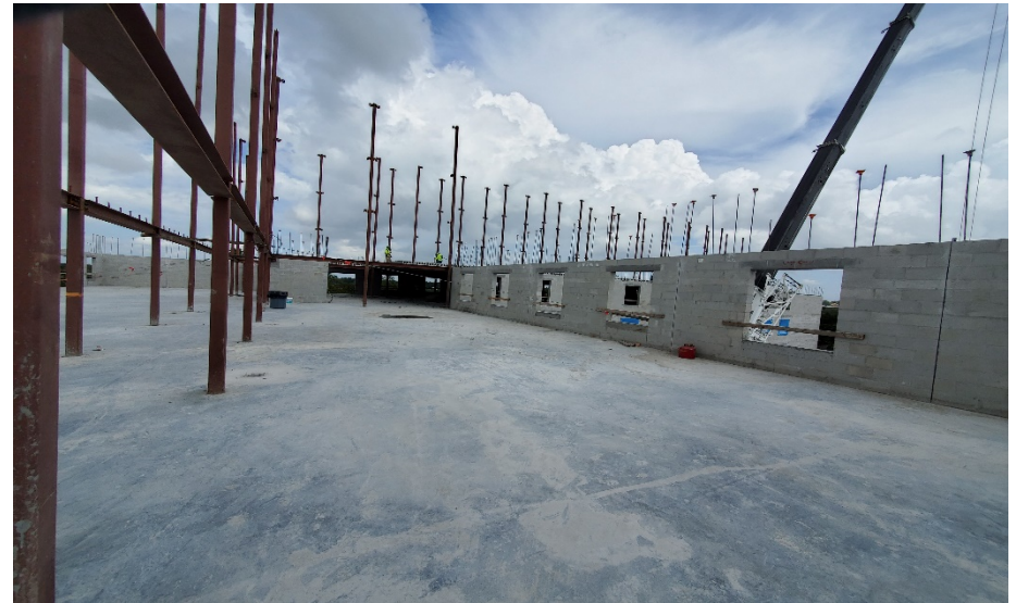
Tower 2 – 7 th Floor Hollow Core Plank Install in Progress
