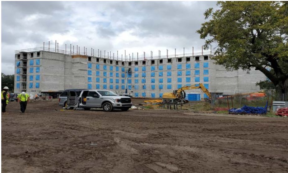
Tower 2 – 6 th to 7 th Floor CMU Walls Install in Progress
