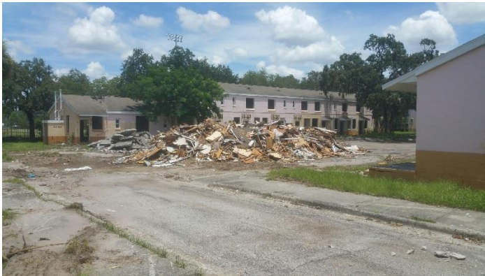
NBH Demo Phase 2 underway.
