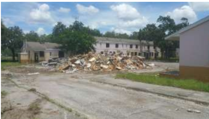
NBH Demo Phase 2 underway.
