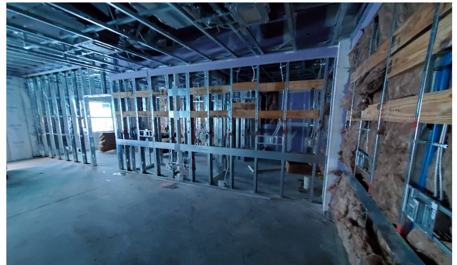
Tower 3 – 3rd Floor Interior Wall Framing in Progress
