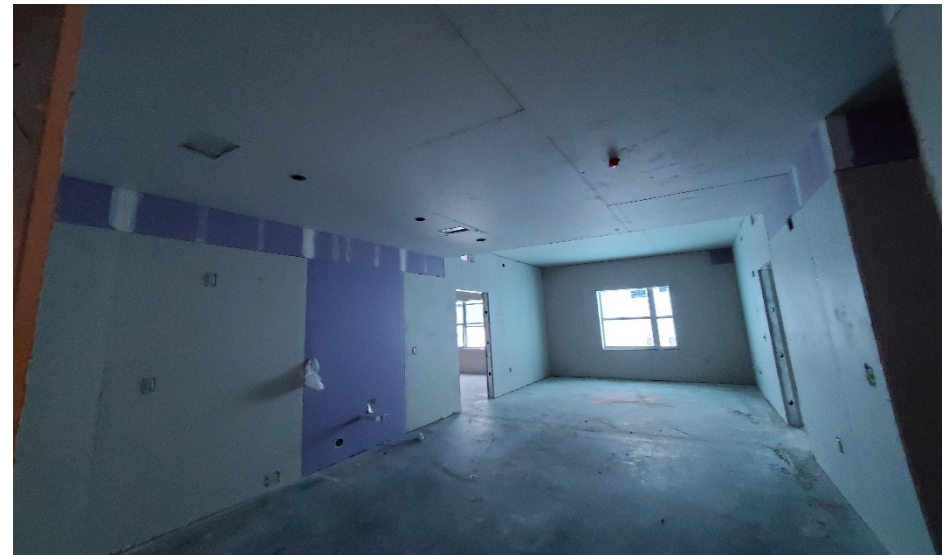
Tower 1 – 1 st Floor Interior Unit Drywall Complete
