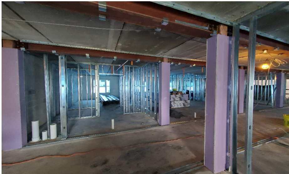
Tower 1 – 4 th Floor Interior Wall Framing in Progress
