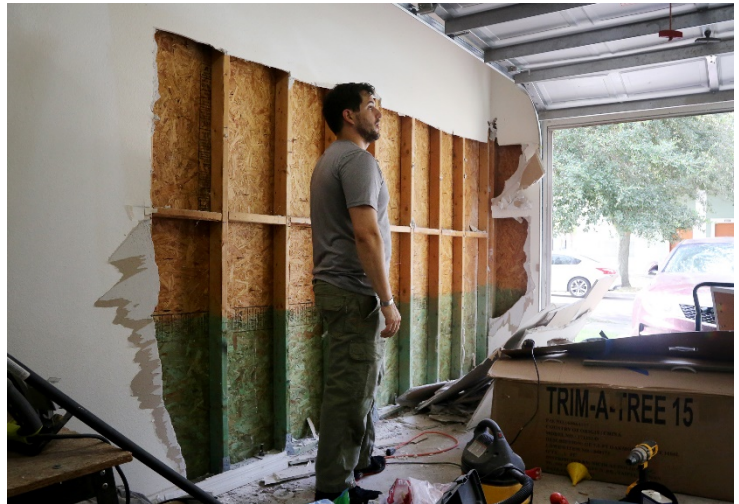
National Guardsman Ryan Steiner, 30, stands in the garage of his home on Machado Street in Tampa. Steiner said he demolished a section of drywall in the garage, at left, to find the manufacturer's stamp so he could identify the origin of the building material. [DOUGLAS R. CLIFFORD | Times.]
