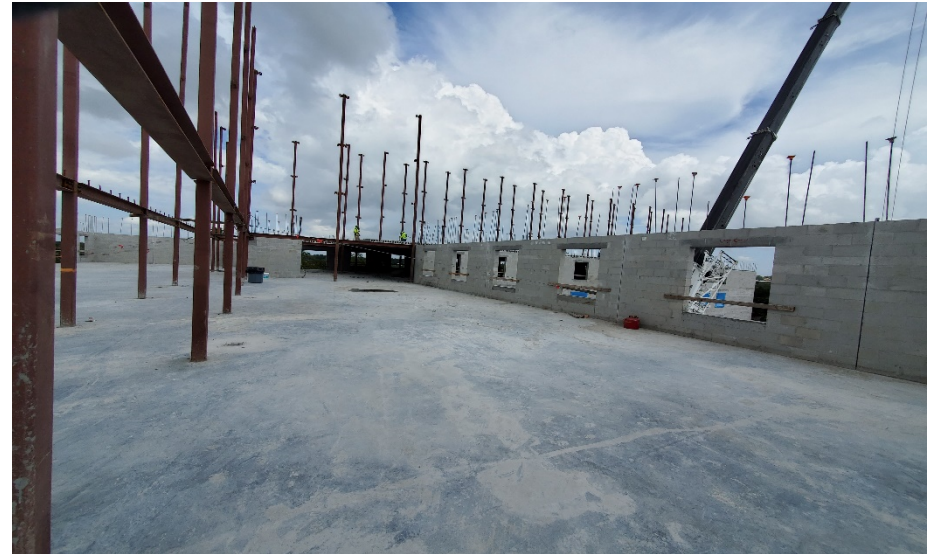
Tower 2 – 6th Floor Hollow Core Plank Install in Progress
