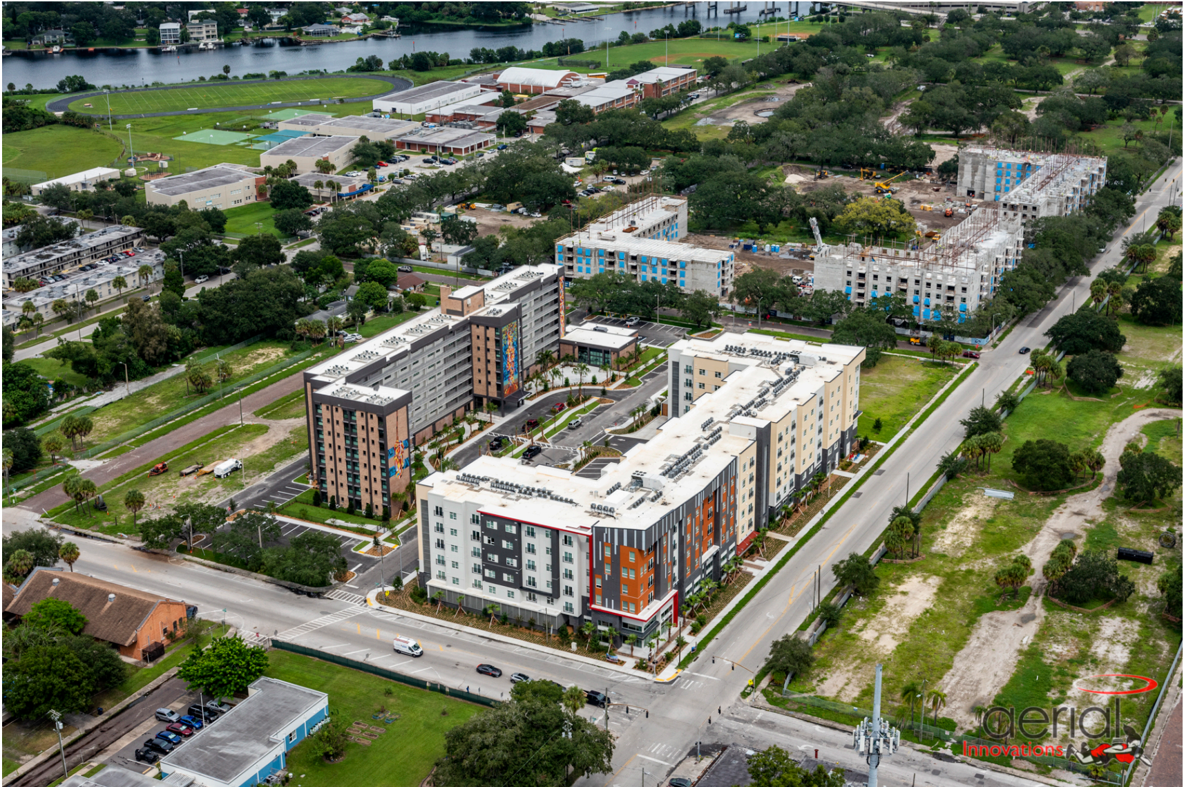
Aerial View of Renaissance, Mary Bethune High Rise, and Boulevard Towers 1, 2, 3, and 4
