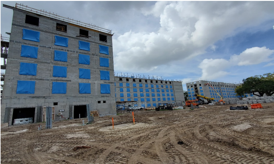
Tower 3 – 6 th to 7 th Floor CMU Walls Install Complete
