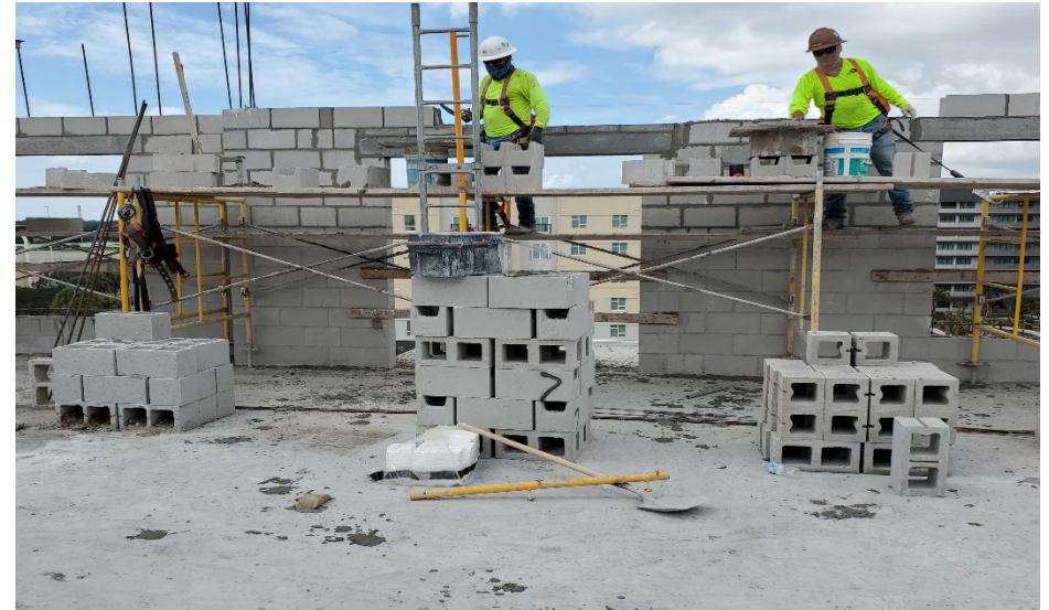
Tower 1 – 7 th to 8 th Floor CMU Walls Install in Progress
