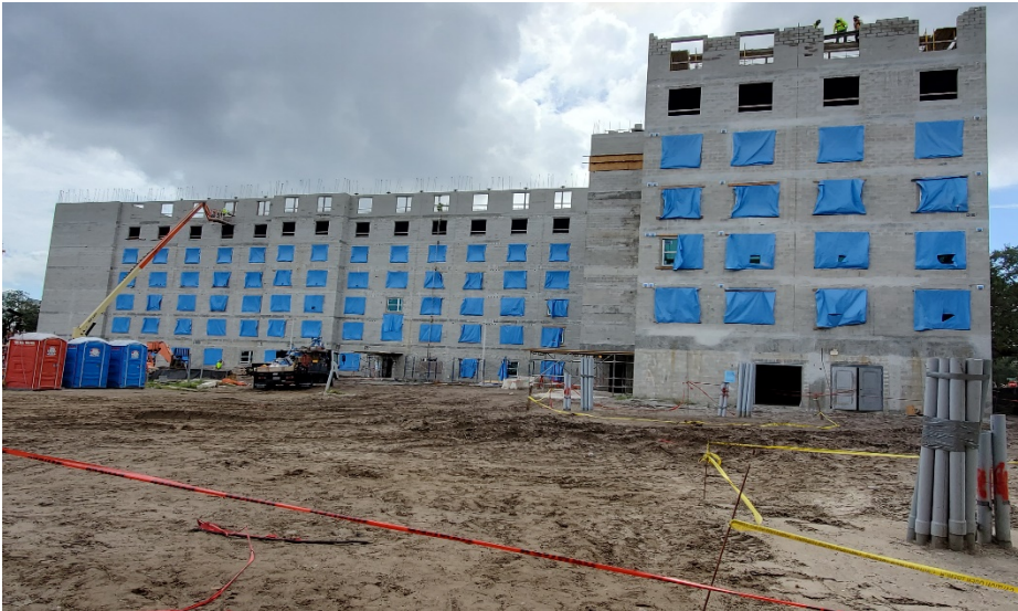
Tower 1 – 7 th to 8 th Floor CMU Walls install in Progress
