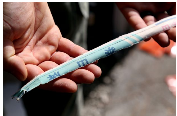
Ryan Steiner holds a strip of paper displaying a manufacturer's stamp that he recovered from a section of drywall on an interior wall in the garage of his home. The drywall tested as toxic. [ DOUGLAS R. CLIFFORD | Times ]
