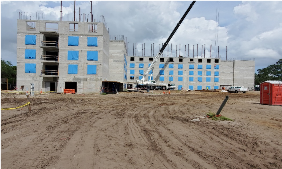
Tower 2 – 5 th to 6 th Floor CMU Walls Install in Progress
