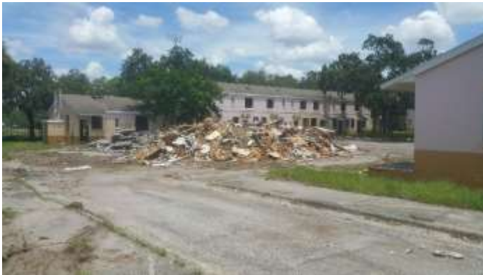
NBH Demo Phase 2 underway.
