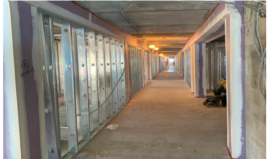
Tower 2 - Interior Framing in Progress
