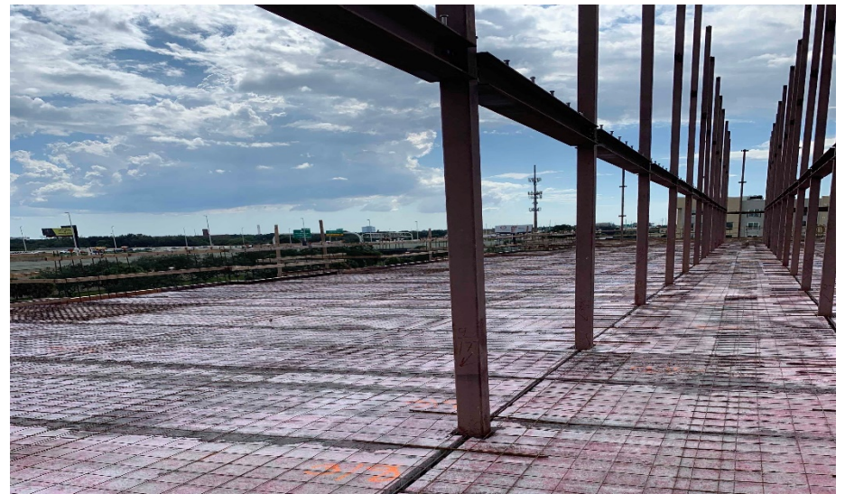
Tower 3 - Hollow Core Plank Installation in Progress
