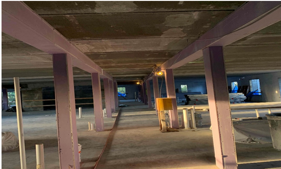
Tower 3 - Support Columns and Beams in Progress
