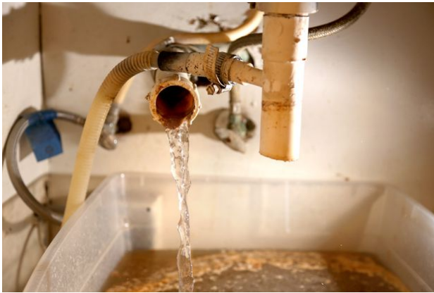
Figure 6 - Water from a kitchen sink drains into a plastic storage tub under the sink of James and Christina Flanning's apartment kitchen. The Flannings say building maintenance workers have avoided repairing plumbing issues, leaving them no option but to discard the water outside. [ DOUGLAS R. CLIFFORD | Times ]
