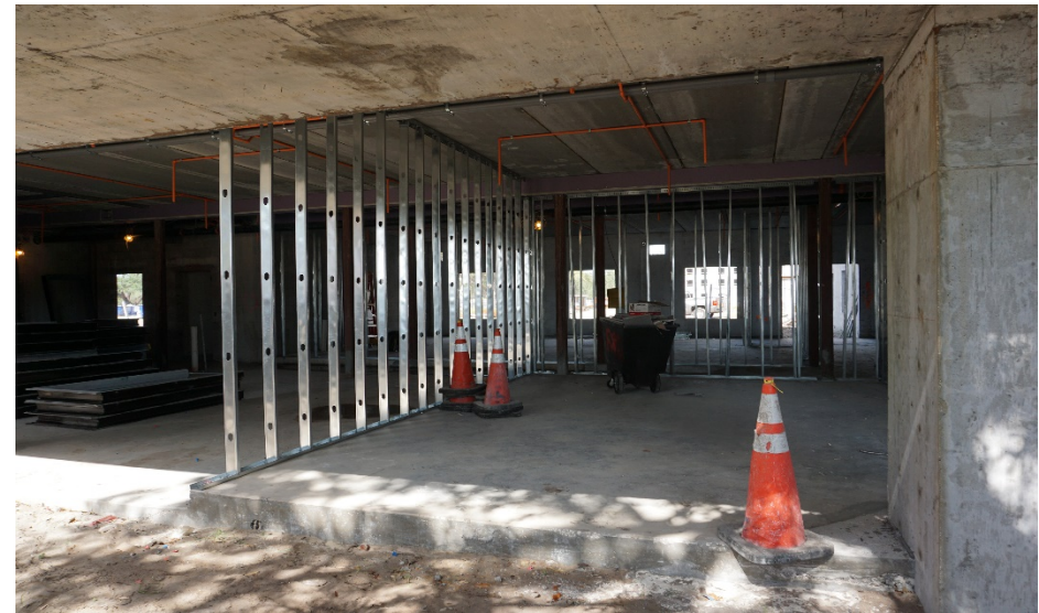
Tower 1 - Interior Unit Framing in Progress
