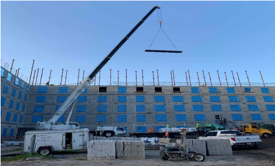
Tower 1 - Hollow Core Plank Installation in Progress
