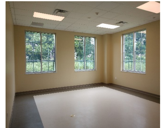
Typical Individual Classrooms
