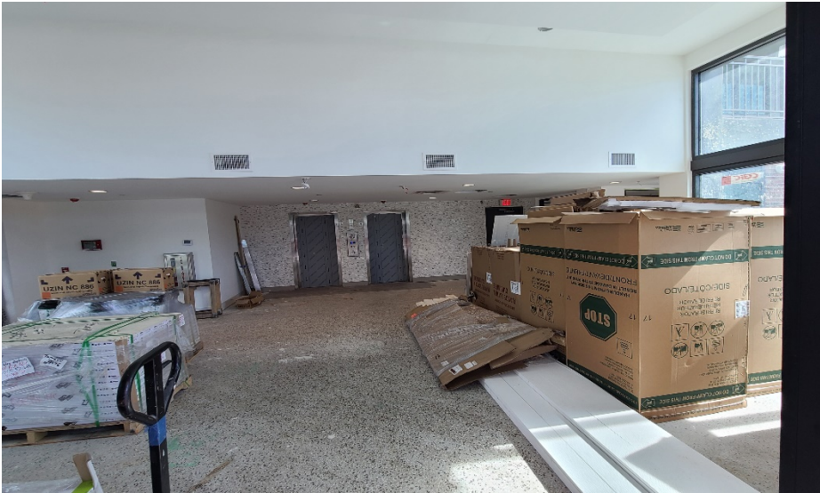
Lobby in Progress
