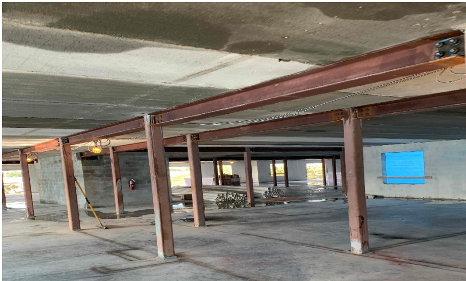
Tower 1 - 1 st Floor Corridor in Progress
