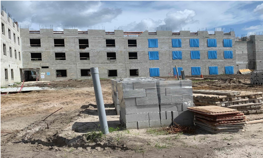
Tower 2 - Exterior CMU Walls in Progress
