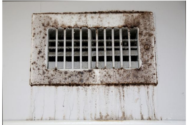
Figure 3 - Mold is visible on an air conditioning vent in the bathroom of James and Christina Flanning's apartment on Monday. James Flanning said he has had to use an inhaler since moving into the apartment. [ DOUGLAS R. CLIFFORD | Times ]
