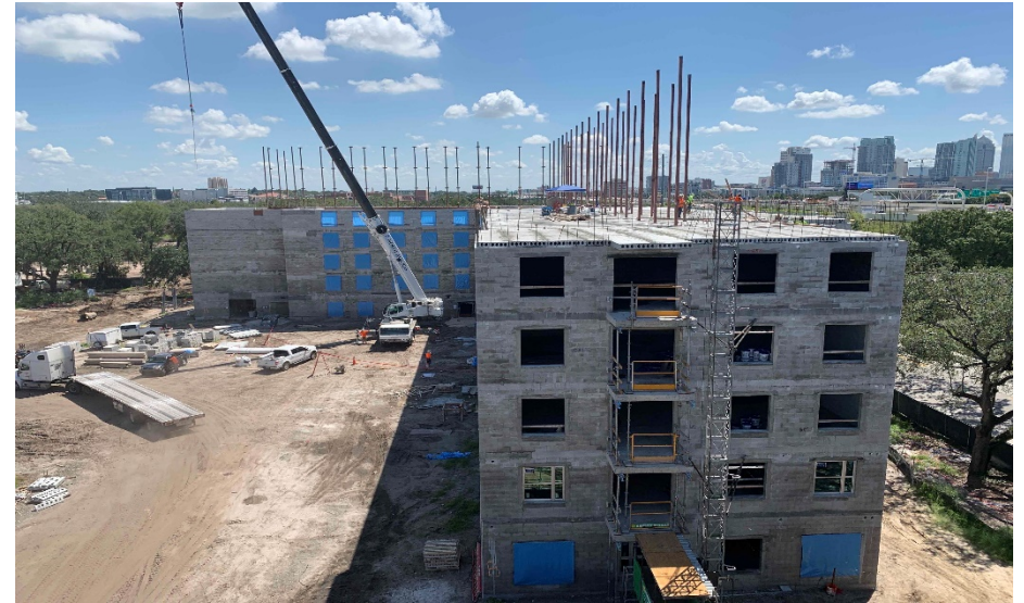
Tower 1 - Hollow Core Plank Installation in Progress
