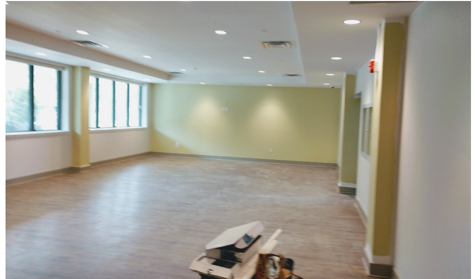
Community Room in Progress
