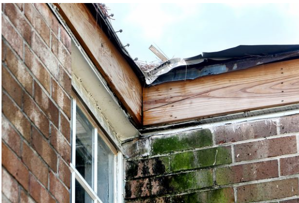
Figure 9 - The exposed wood and damaged fascia of a Timberfalls apartment building. [ DOUGLAS R. CLIFFORD | Times ]
