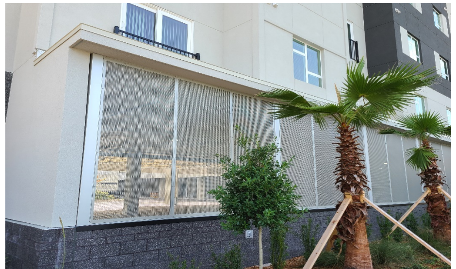
Parking View from Rome Avenue
